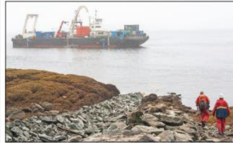
Above, a Westpark Electric crew moves between shore and barge on Thursday during installation of a fiber-optic cable at Mountain Point. The barge Empire 45 arrived early Thursday morning with tugs Arctic Tug and Island Tugger. Crews connected the cable from Prince Rupert to Ketchikan at a recently constructed communications hub at Mountain Point. Fiber-optic cable was unraveled from a large orange spool located at mid-ship and was fed off the stern of the barge.
