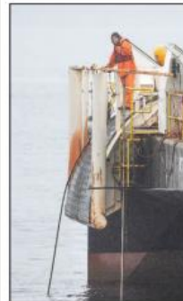
Above, a Westpark Electric crew moves between shore and barge on Thursday during installation of a fiber-optic cable at Mountain Point. The barge Empire 45 arrived early Thursday morning with tugs Arctic Tug and Island Tugger. Crews connected the cable from Prince Rupert to Ketchikan at a recently constructed communications hub at Mountain Point. Fiber-optic cable was unraveled from a large orange spool located at mid-ship and was fed off the stern of the barge.
