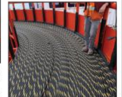
The submarine fiber-optic cable is shown spooled aboard the barge Empire 45.
